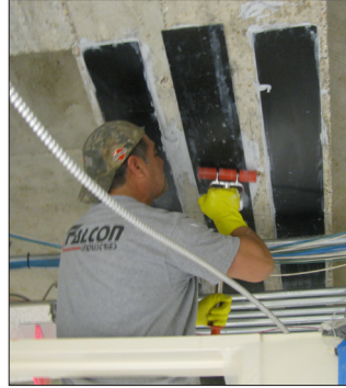
Applying CFRP strips to underneath of beam
