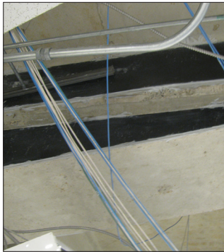
Shear plates on side of beam
