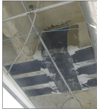
U strip applied to beam
