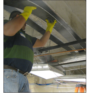
Threading CFRP strip over duct work
