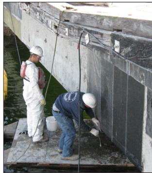
Applying CFRP fabric for shear strengthening
