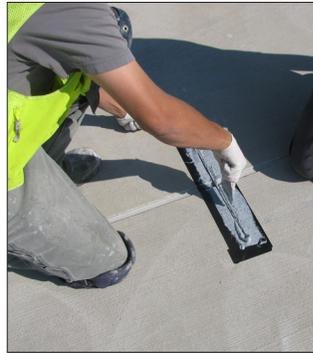
Inserting biscuit in slot
