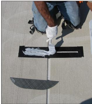
Applying epoxy paste to slot
